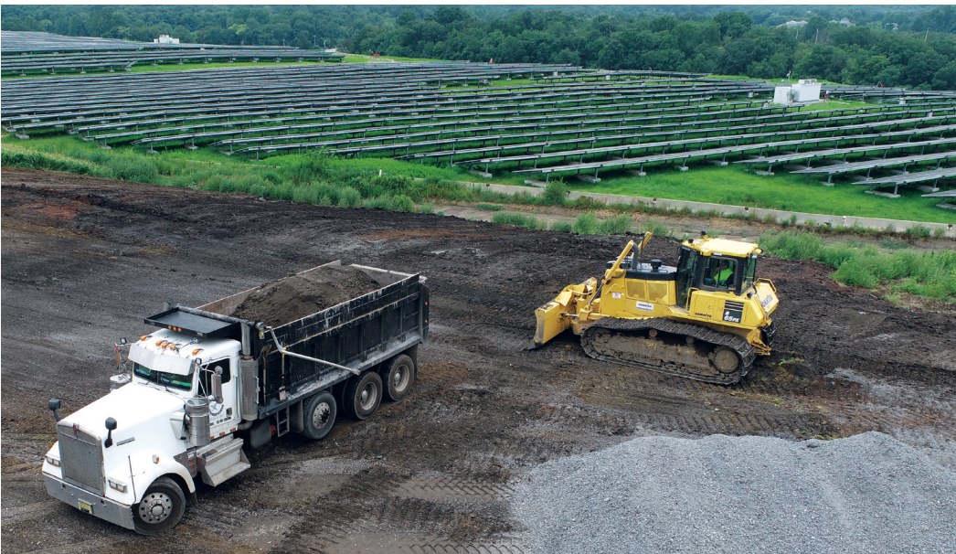
Materials delivered by truck are graded to eliminate low areas where stormwater collects and infiltrates.
