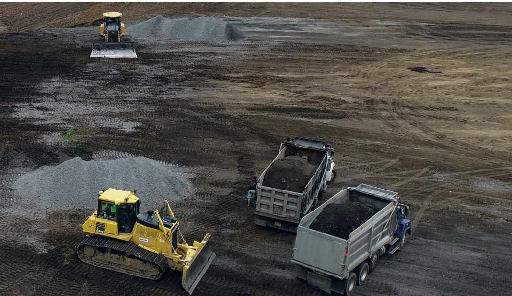
The regrading program restores slopes to conditions optimal for promoting stormwater runoff while directing the runoff to existing on-site stormwater controls.
